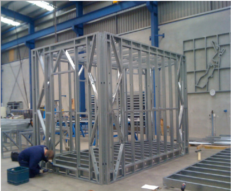
Figure 44 - Architectural module in construction
