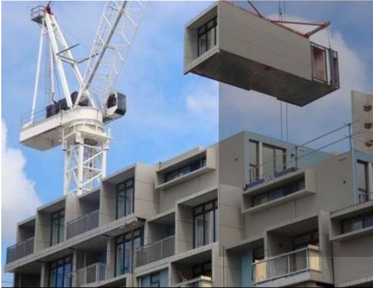
Figure 43 - Architectural module stack up
